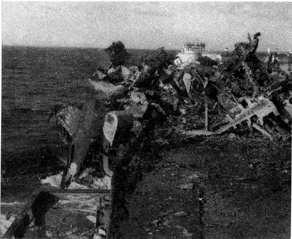
Clearing away the foamite and wreckage, May 4 1945
