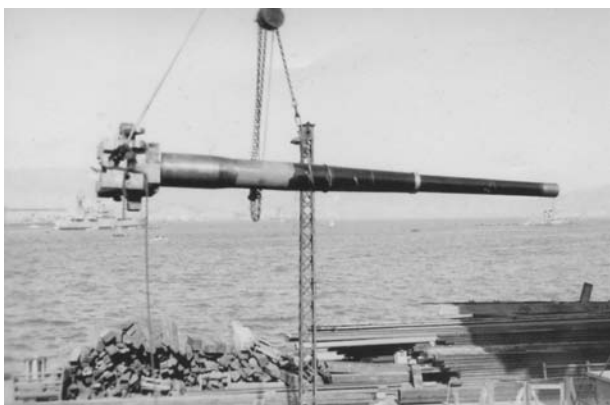
Replacement of 4.5" X Gun , by Anti Submarine Mortar system
