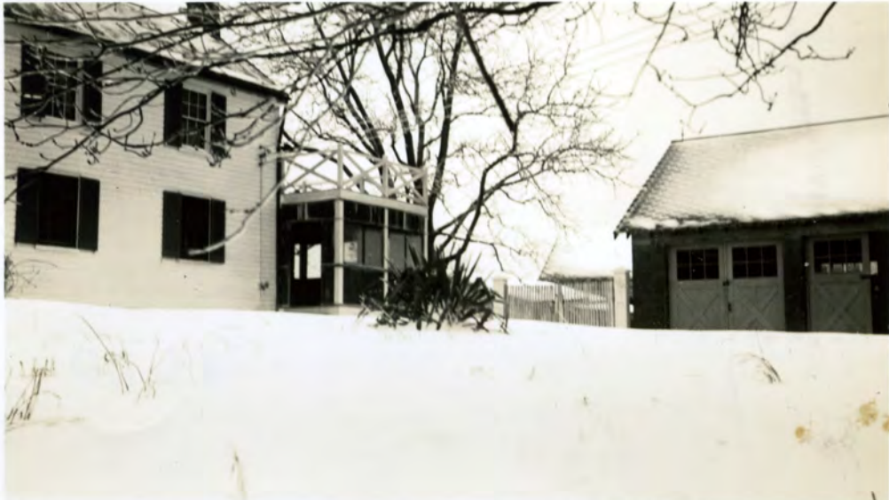
side of house - entrance to Garage & Kitchen
