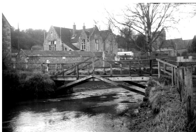
Figure 4. – Footbridge & river Wylfe at Longbridge (1964). Church and school ('faith' & 'hope') in the background.
